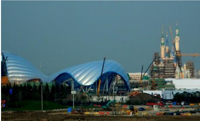
Construction workers in December 2015 at Shanghai Disney Resort. Photo: CFP
